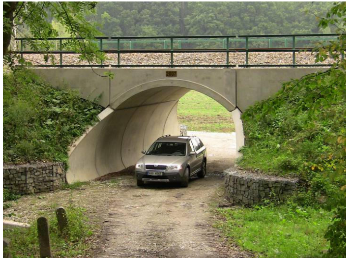
The new bridge
